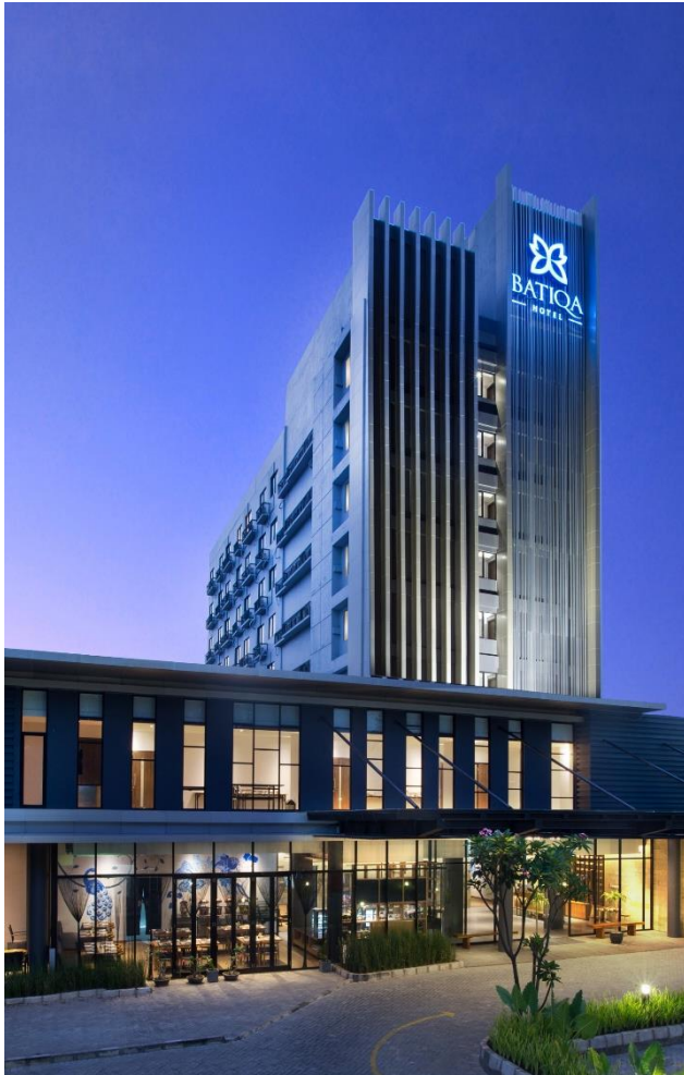
Exterior view of BATIQA Hotel Cirebon
